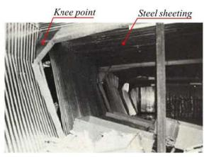
(b) Collapse that took place during the winter of 1976/77 in Sweden (Jchannesson & Johansson, 1979). The three hinged portal steel frames were stabilized laterally by use of a corrugated steel sheet (diaphragm action) that was assembled on top of the frames.
