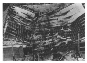
(**b**) A picture taken after the collapse. Note that there is no visible braced bay.
